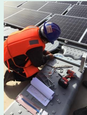
4 Connecting the PV floating arrays together and securing to the mooring system
