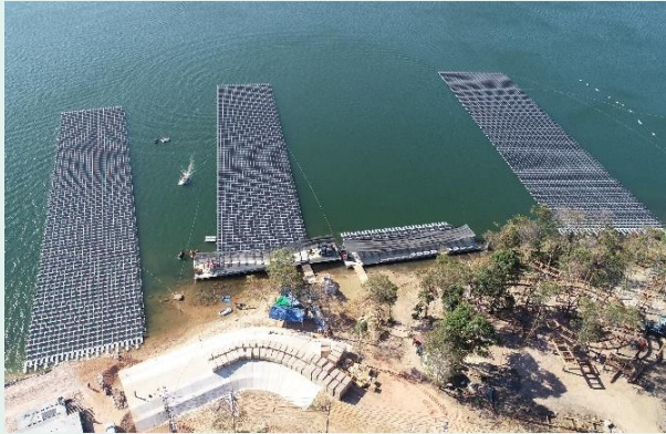
3 Moving the PV floating array to the installation area
