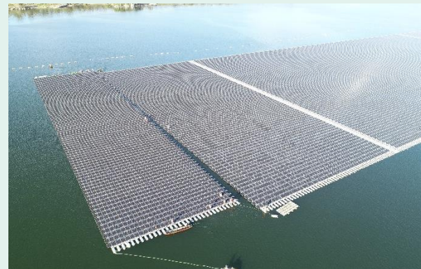
4 Connecting the PV floating arrays together and securing to the mooring system
