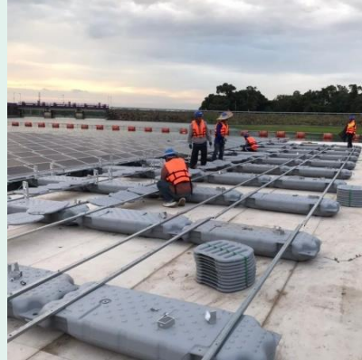
4 Connecting the PV floating arrays together and securing to the mooring system
