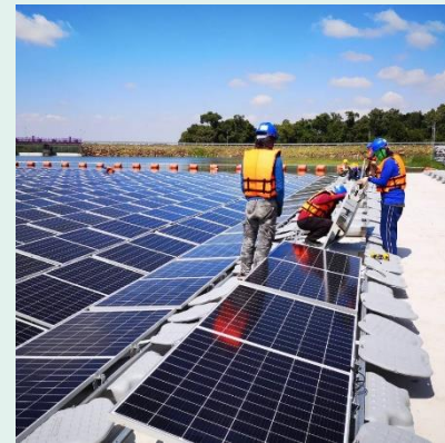
4 Connecting the PV floating arrays together and securing to the mooring system
