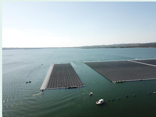
4 Connecting the PV floating arrays together and securing to the mooring system
